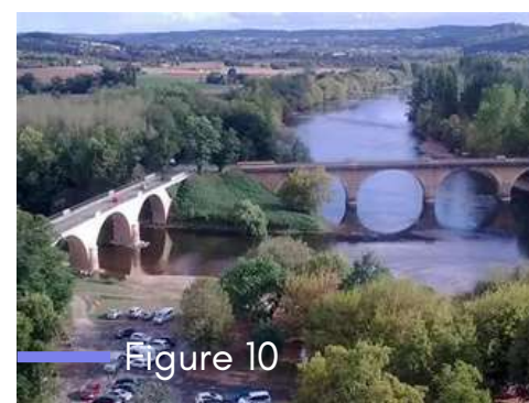
Figure 10 ponts de Limeuil
